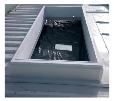
4. Special Aluminium L profiles must be positioned and fixed around upstand. Position of this L profiles is on the location of the holes on the glass unit.
