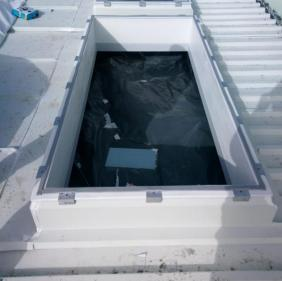
6. Glass unit must be positioned and pressed down, then must be screwed all around from the side (picture below)
